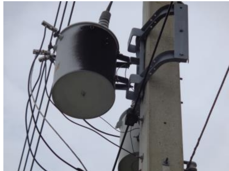
Photo 12: View of the pole-mounted transformer to the west of the site along N Magnolia Ave.
